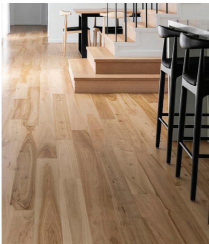
Residential Home, Queensland This architect designed two storey luxury home features 140mm x 15mm Blackbutt hardwood flooring, finished with Bona Traffic Matt.
